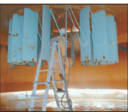
A technician cleans lime deposits from impellers at the City of Sunrise (Fla.) water treatment plant, using a 40,000 psi rotary gun.
