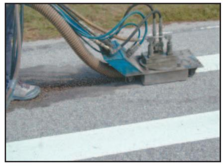
A technician removes a 6-inch thermoplastic highway stripe using Precision Hydroblasting's custom-designed floor machine, operating at 40,000 psi/4 gpm. The unit has 12 nozzles, two 6-inch spray bars, and vacuum containment.
